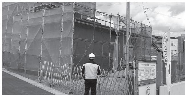
(社屋新築工事)
