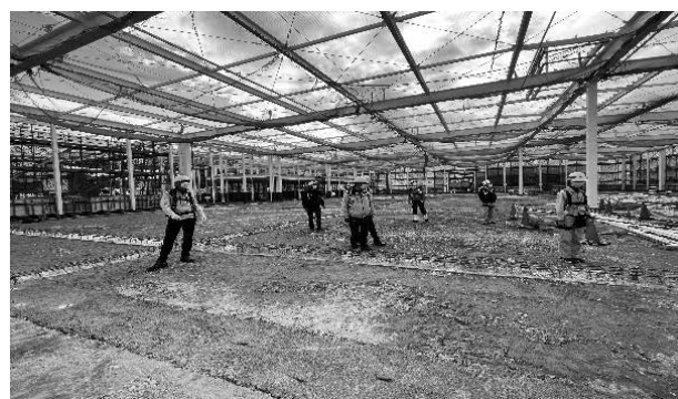
工場新築工事
